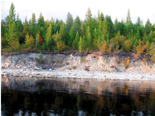
Fig. 8. Thermoabrasion right bank of Vilyui Reservoir in Section No. 7 near mouth of Ust'-Chon "pipe" composed of highly weath-
